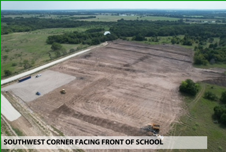
PREPARING SITE FOR NEW PAVING AND BUILDING FOUNDATION
