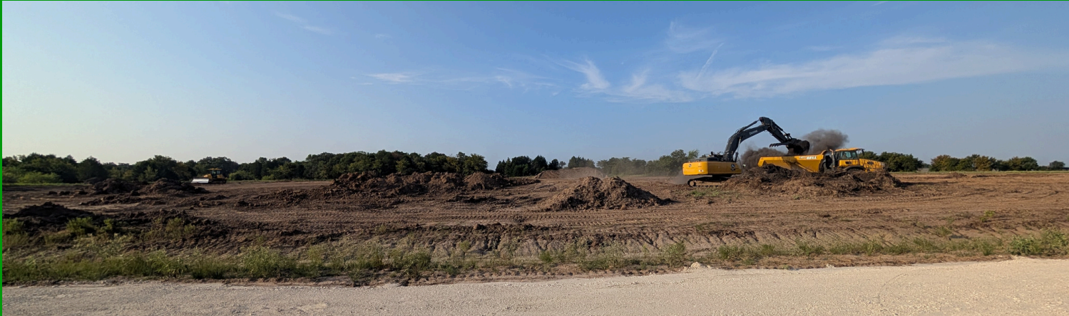
PREPARING SITE FOR NEW PAVING AND BUILDING FOUNDATION
