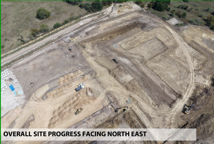
MAIN ENTRY DRIVEWAY IS BEING CUT IN AND COMPACTED
