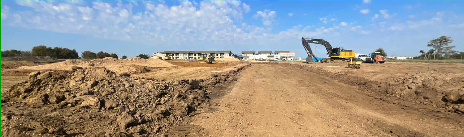
MAIN ENTRY DRIVEWAY IS BEING CUT IN AND COMPACTED
