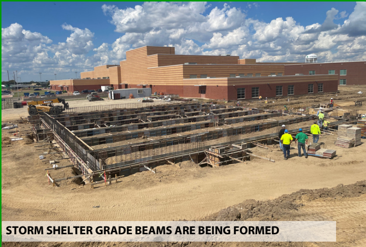
OVERALL PROGRESS OF BUILDING ADDITION
