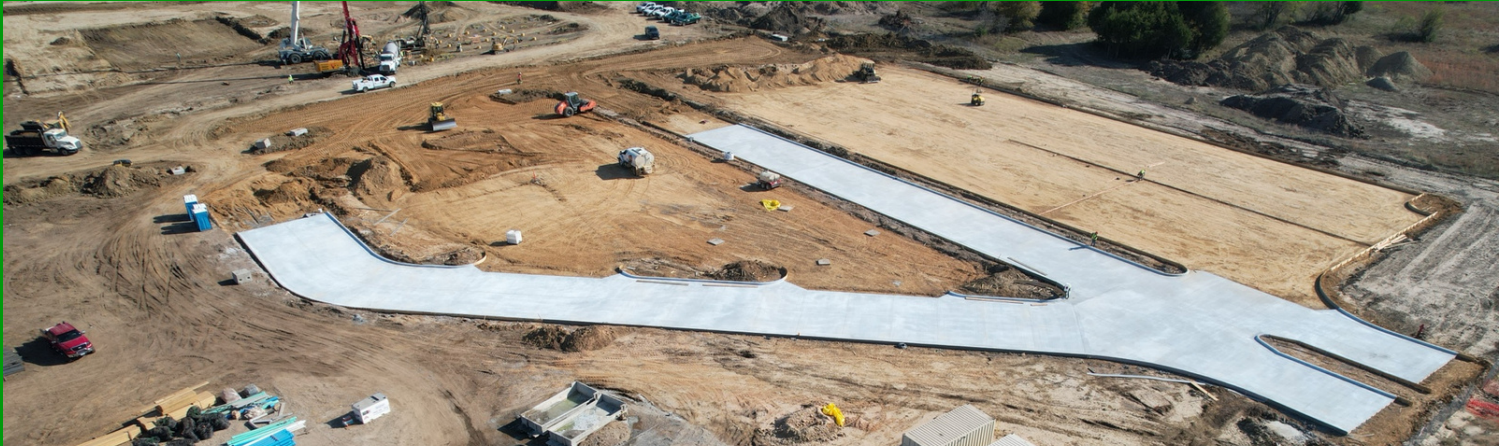
MAIN ENTRY DRIVEWAY HAS BEEN PAVED AND SELECT FILL IS BEING INSTALLED IN THE PARKING LOTS
