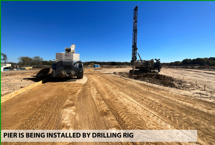
OVERALL BUILDING FOUNDATION PROGRESS
