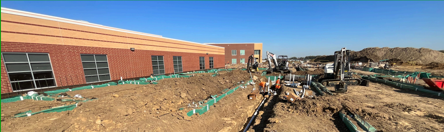
INSTALLATION OF BUILDING FOUNDATION GRADE BEAMS CONTINUES
