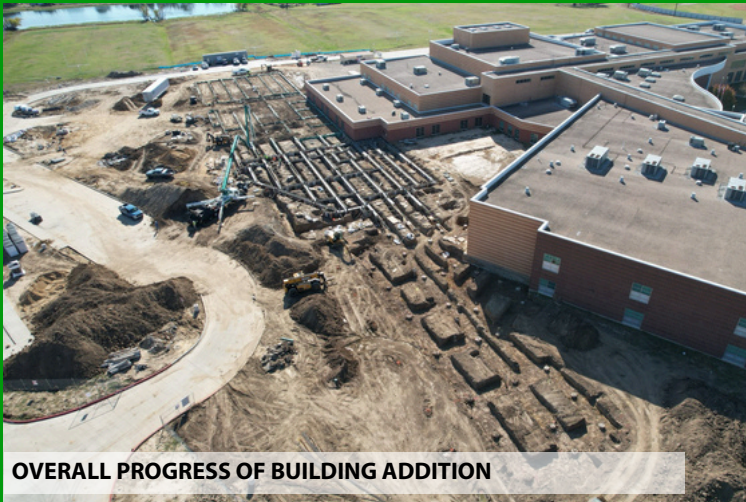
INSTALLATION OF BUILDING FOUNDATION GRADE BEAMS CONTINUES
