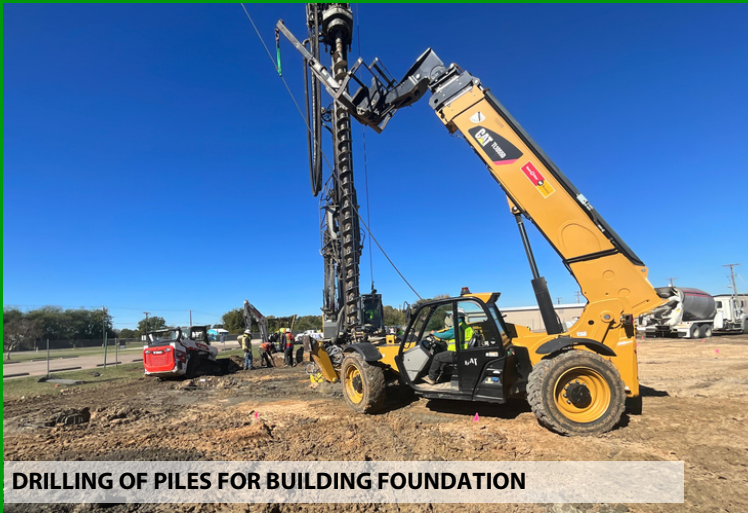
OVERALL PROGRESS OF CLASSROOM ADDITION (STORM SHELTER) FOUNDATION
