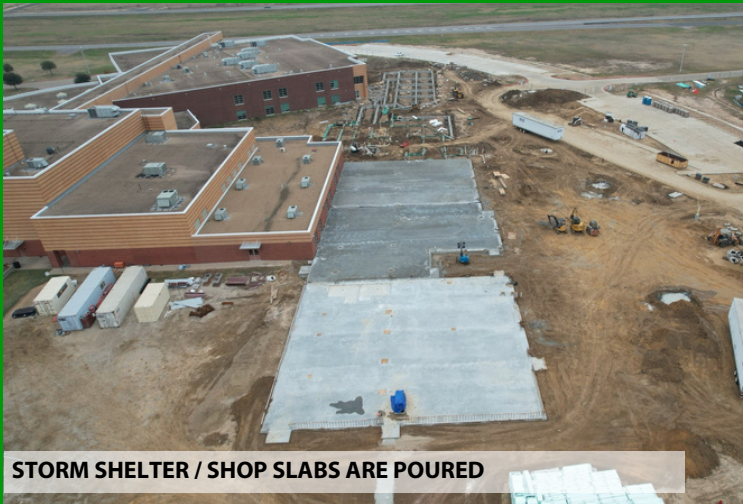
OVERALL PROGRESS OF CTE ADDITION
