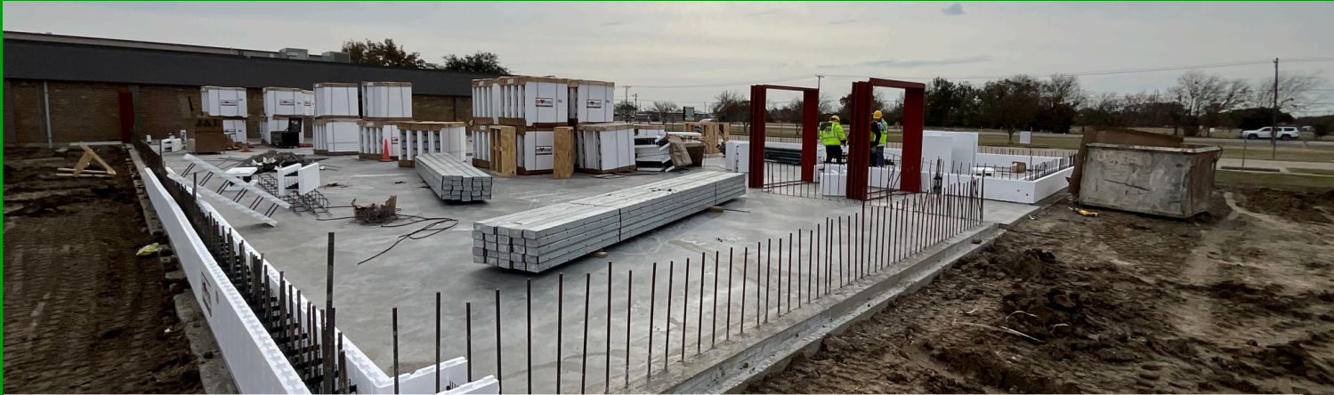
GRADE BEAMS ARE BEING WRAPPED & PREPARED FOR SLAB POUR
