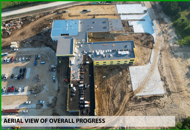
OVERALL PROGRESS FACING NORTHWEST
