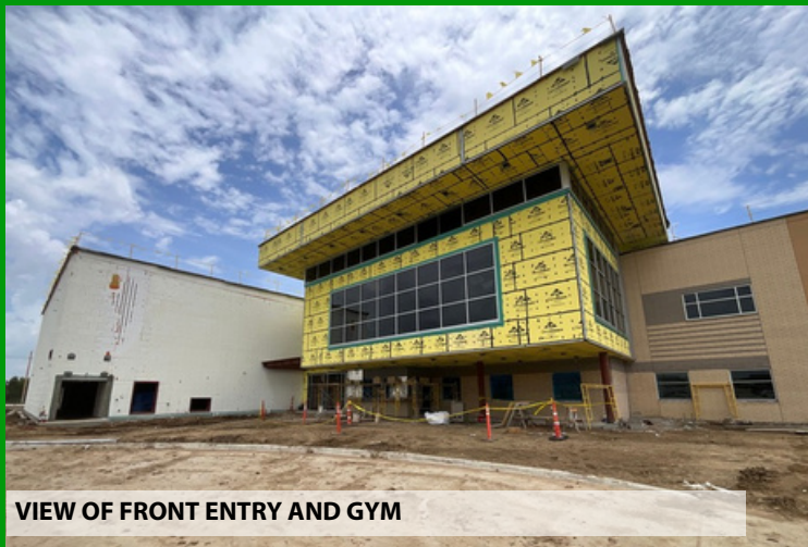
OVERALL PROGRESS LOOKING EAST
