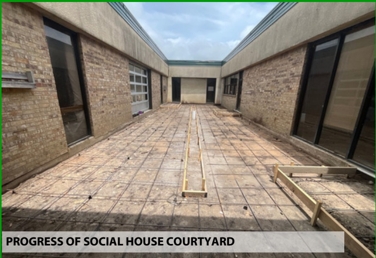
PROGRESS OF CAFETERIA RENOVATION
